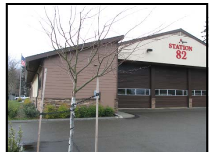
S82 Bay Doors on opposite side of station as conference room
